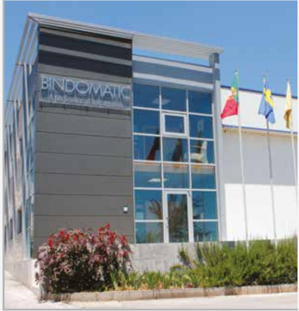
Bindomatic Portugal facilities, in Loureira.
